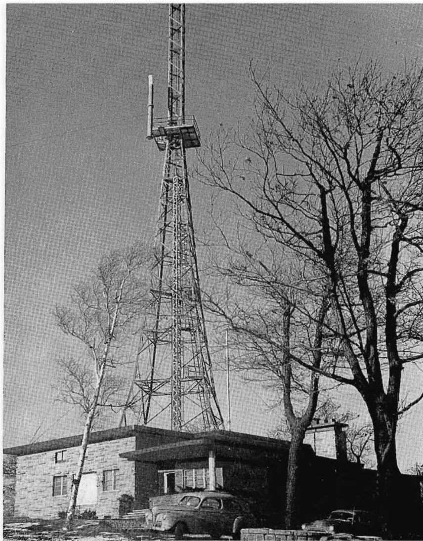
FIG. 3. Two-section heavy duty Pylon passing microwave platform. Constant cross-section of tower from this point to the top is for channel 6 Supergain Antenna.
